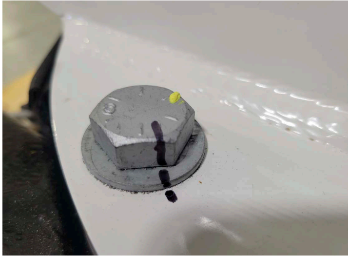
Figure 3-7. Marking Bolt Heads Prior to Torque Check
