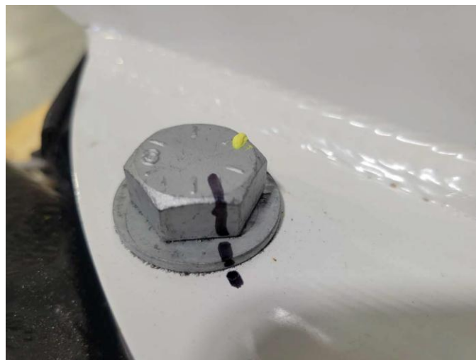
Figure 3-7. Marking Bolt Heads Prior to Torque Check
