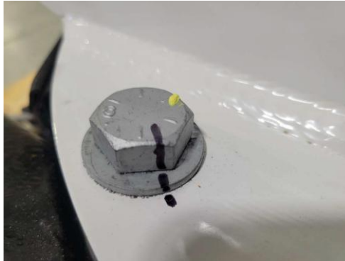
Figure 3-7. Marking Bolt Heads Prior to Torque Check
